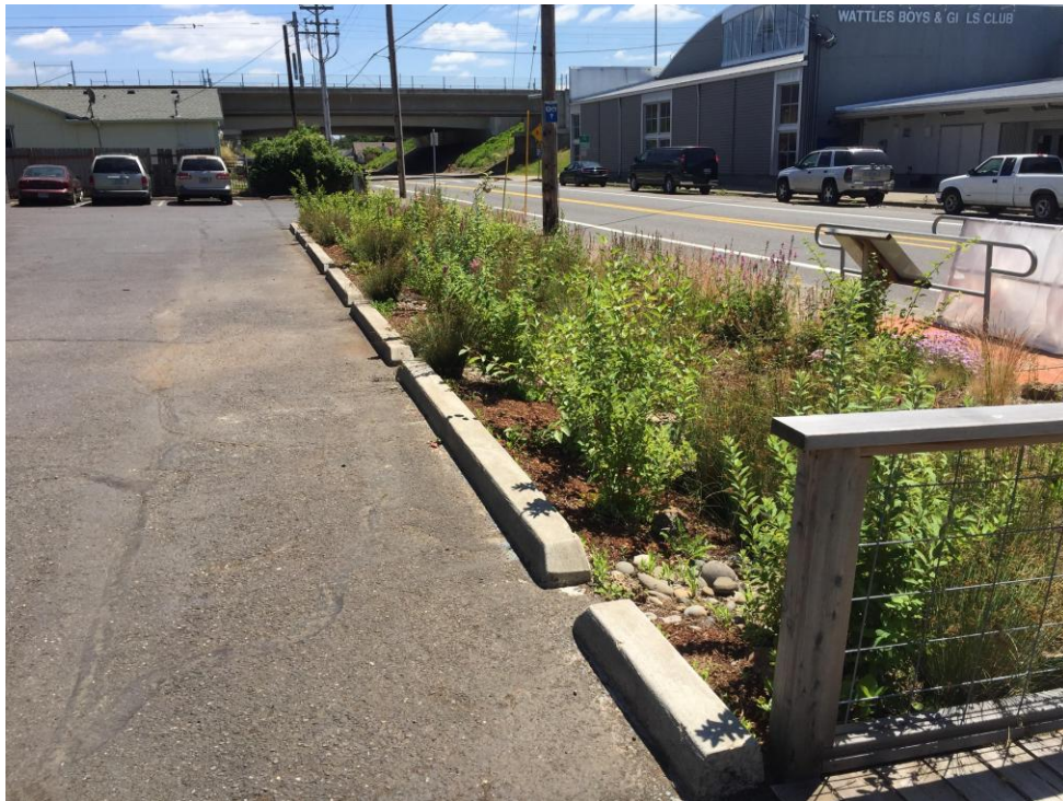
Figure 7. Examples of Bioretention BMPs and a Permeable Pavement System
